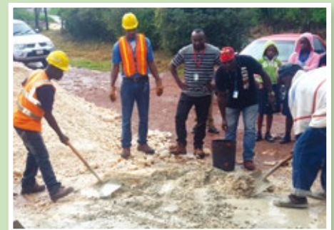
Volunteers from Jamalco paving a road at Campbell's Castle Primary School
